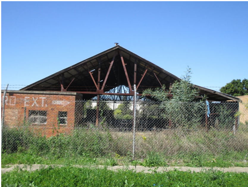
02 - View of existing structure on site
